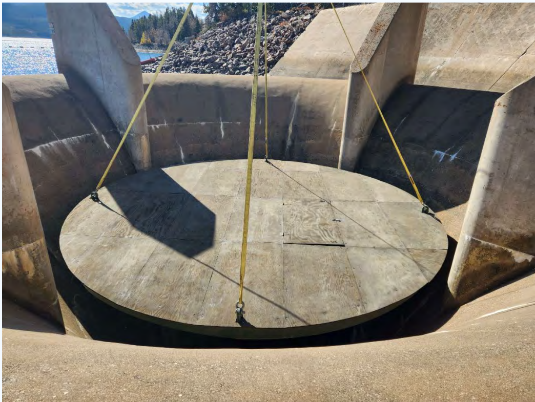
Every fall, Denver Water crews place a 6-ton steel plug into the Morning Glory spillway
