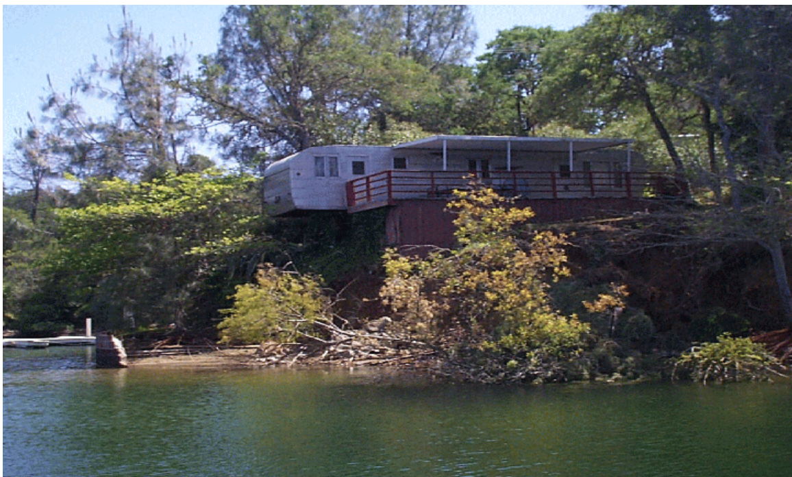
Figure 2. A mobile home extending over the embankment because of erosion at Lake Berryessa. (Office of Inspector General photograph)
