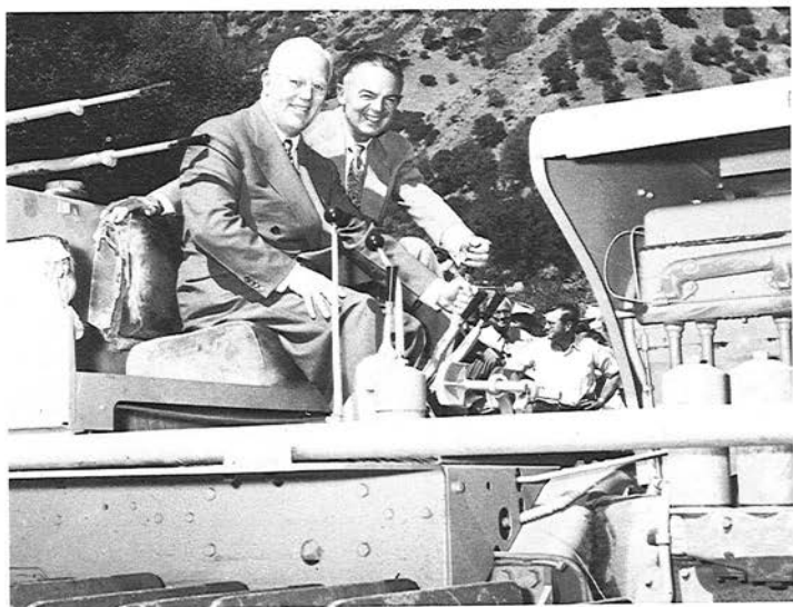
Governor Earl Warren and State Senator Luther Gibson Break Ground for Construction of Monticello Dam in 1953
