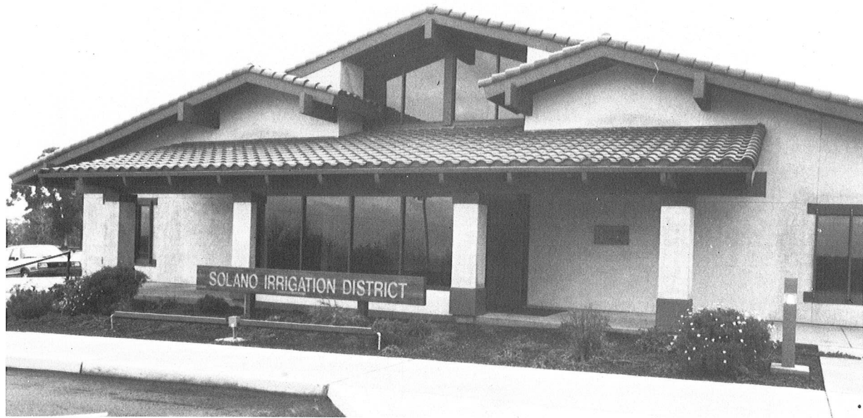
S.I.D.'s Award Winning Offices, Completed in 1985
