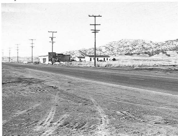
Main Street After Most of the Clearing Had Been Done
