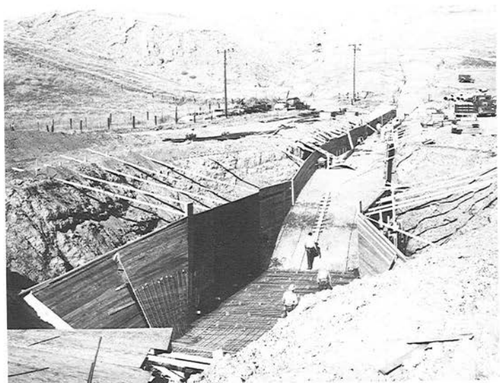
Construction of the Putah South Canal
