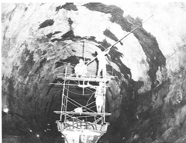
Interior of the Spillway Tunnel
