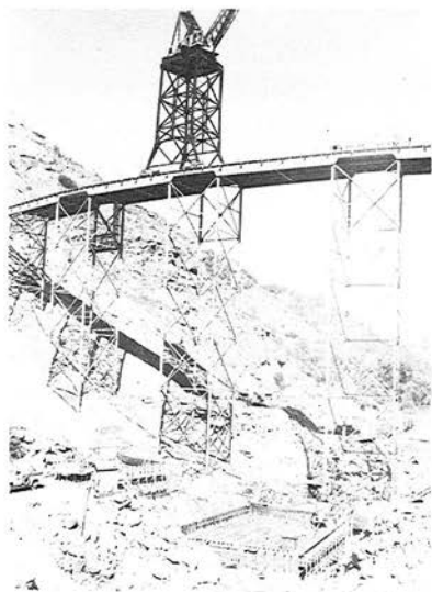
General View of the Concrete Placing Operations
