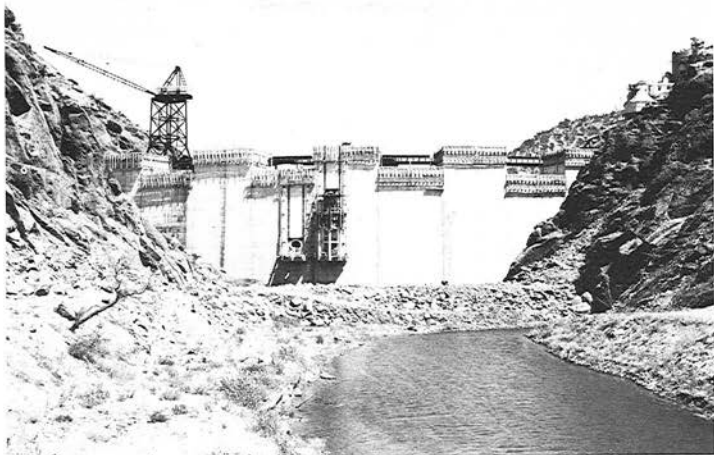
Lakeside Face of Monticello Dam
