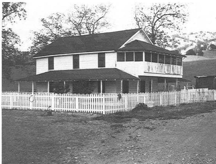
Original Scribner House in Monticello Before its Relocation
